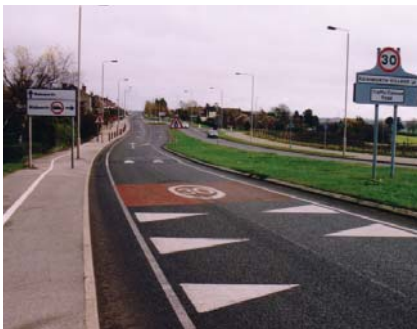
Road hump with no speed reducing feature at the start. Keith Sharples Photography.
